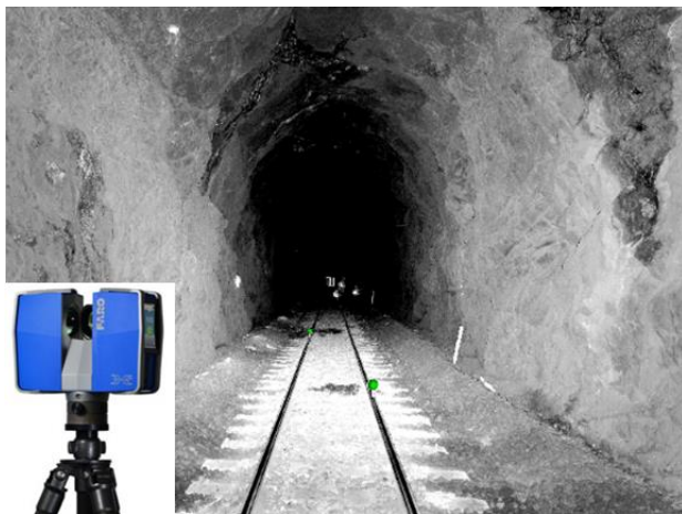
Figure 1. Faro Focus 3D Laser Scanner (Faro Inc.) and an example of the TLS tunnel image (point cloud) generated by this instrument.
