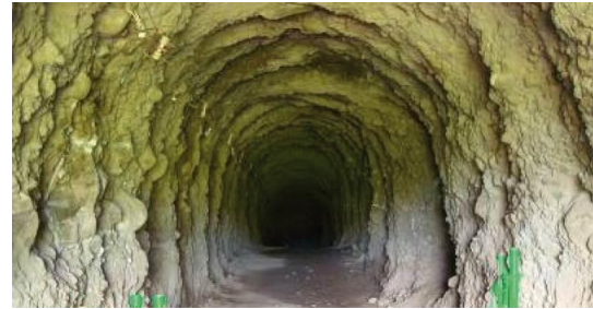
Figure 2. Example of an investigation tunnel.
