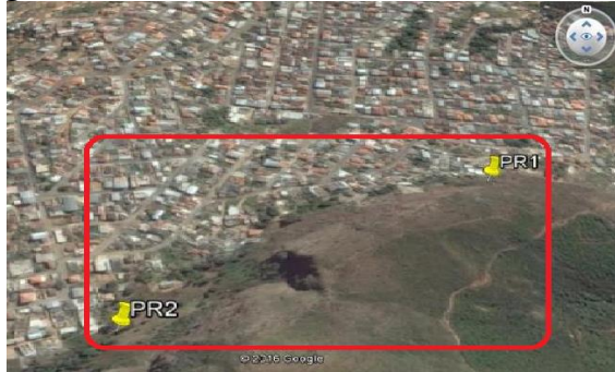
Figure 1: Geographic location of the rock slope, showing the survey points (Google earth).
