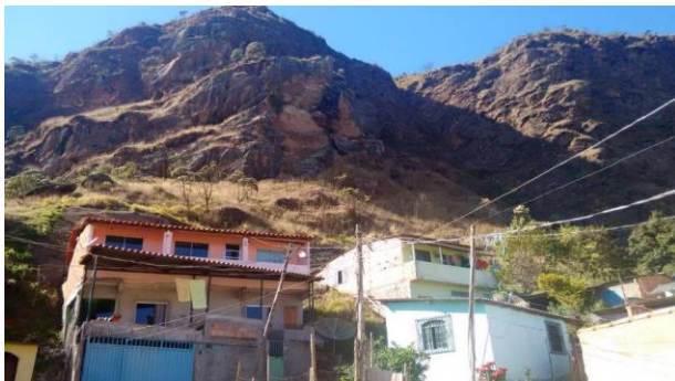
Figure 2. Slope in the Cabanas district.
