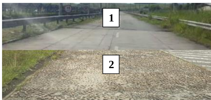
Figure 3. Pista Senoidal e Pista Granulosa
