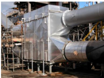
Figura 5. Thermosyphon heat exchanger.
