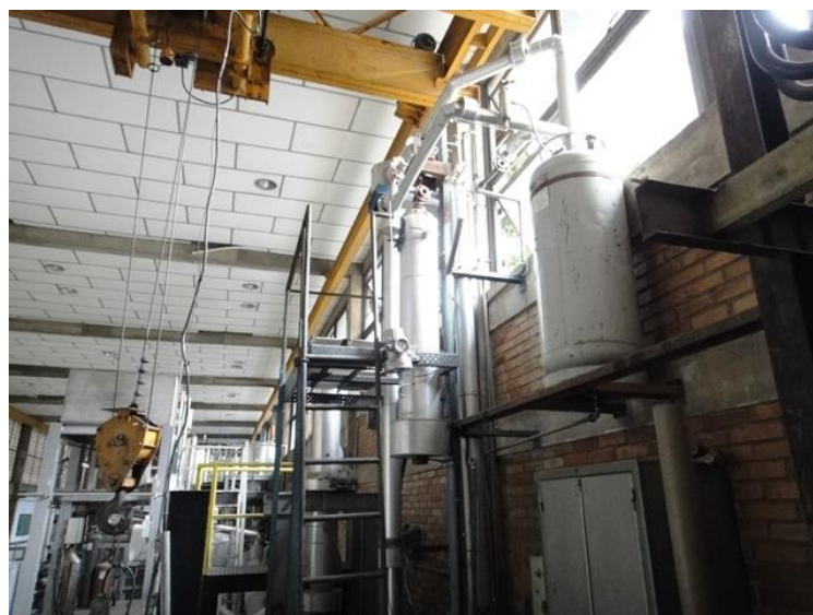
Figure 1. Test Facility for Rewetting (ITR)
