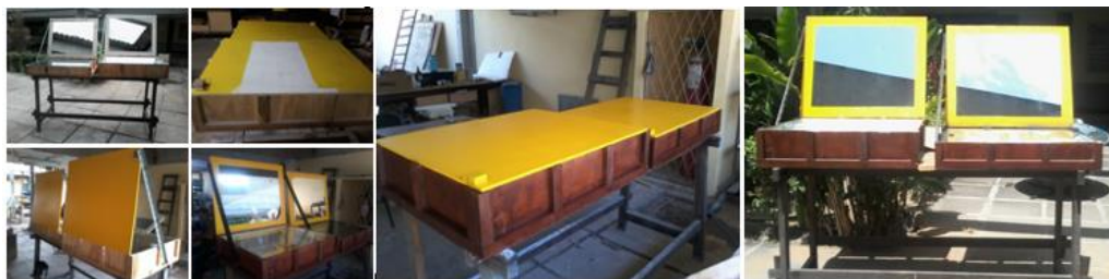
Figure 3. Last steps of the construction of the ovens.
