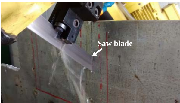
Figure 6a. Cutting the support.
