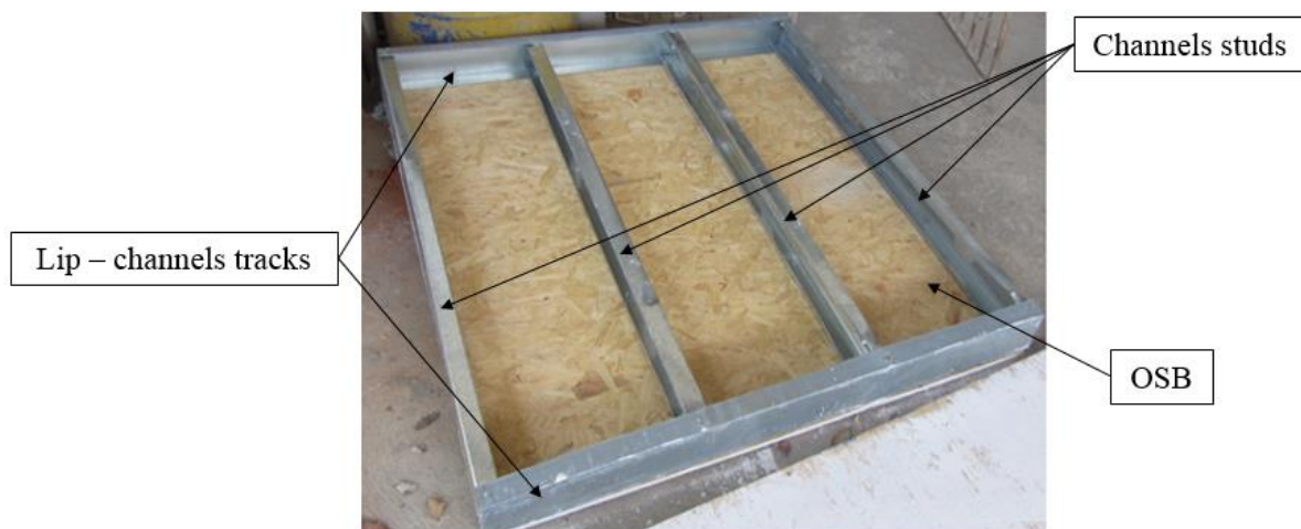
Figure 1. Small LSF wall without one of the OSB covering faces (NUNES, 2017)
