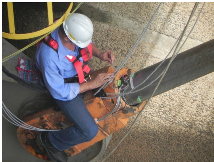
Figure 3. Strain Gages Installation
