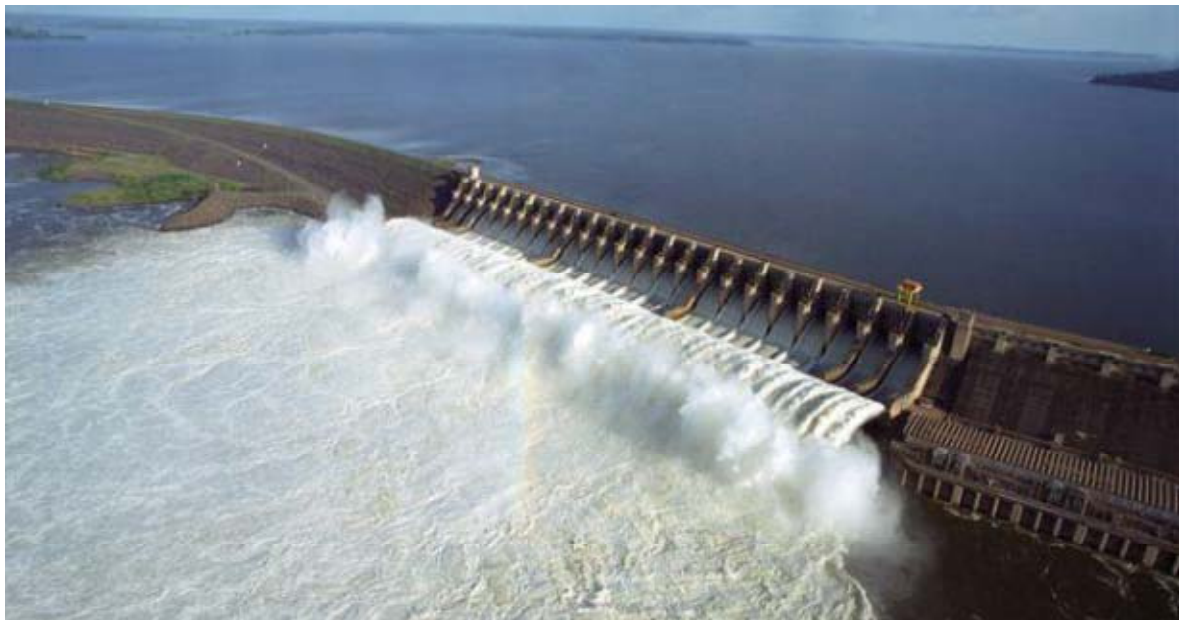
Figure 1. Spillway of HPP Tucuruí
