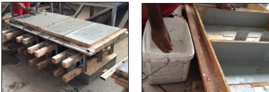
Figure 16 – Pouring concrete 2 nd step and application of grease
