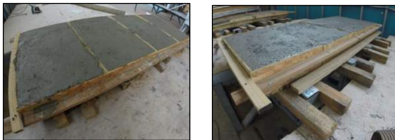
Figure 15 – Pouring concrete 1 st step
