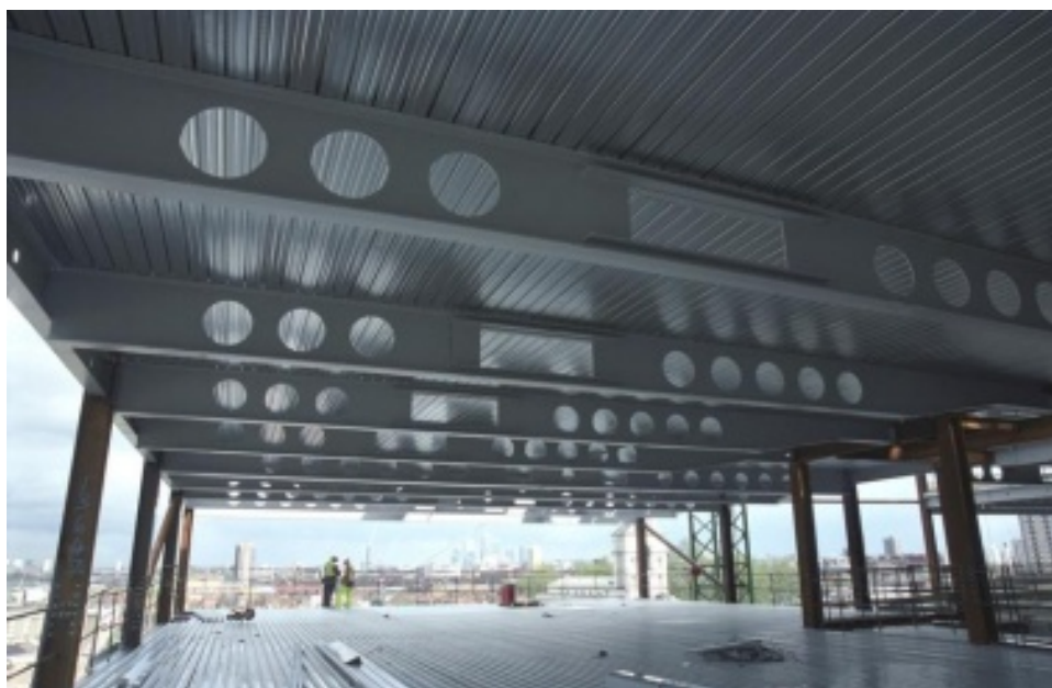
Figura 1 – Vigas mistas com aberturas na alma (steelconstruction.info, 2017)
