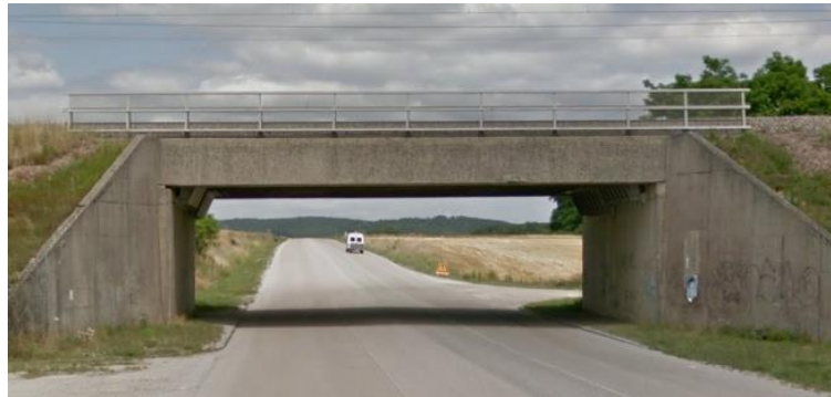
Figure 8. PK 075+317 Viaduct on the Paris-Lyon high speed train track
