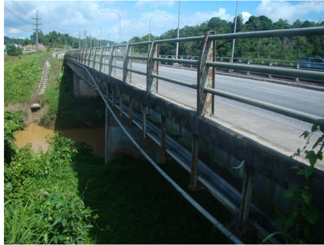
Figure 1. Bridge over the Sebiu river
