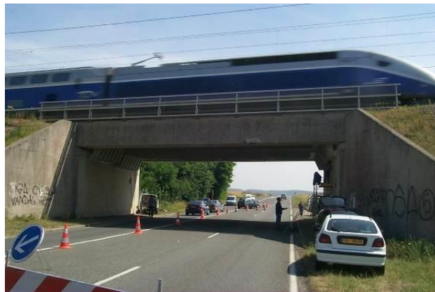
Figure 3. Side view of viaduct.
