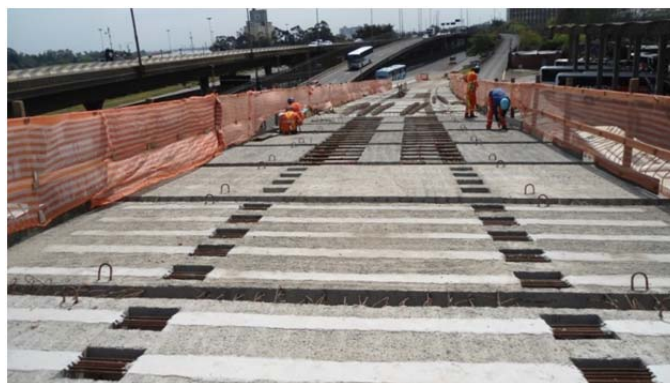
Figure 6. Shear Pockets of Prefabricated Concrete Slabs
