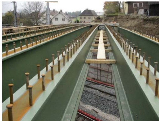
Figure 4. Welded Shear Connector Stud Bolts
