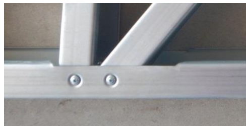
Figure 1 – Bracing and diagonal connected to the chord with self-drilling screws.
