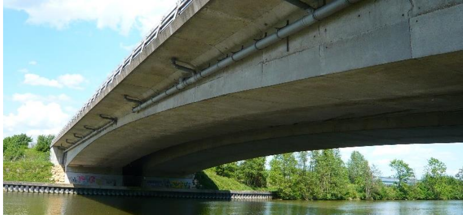
Figure 10. PI-57 Bridge, France.
