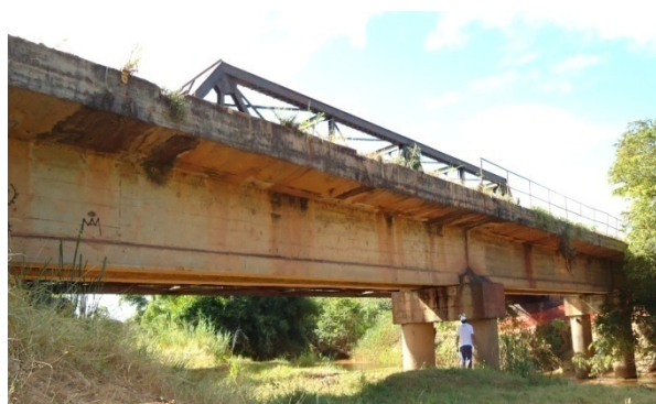
Figure 11 - Oblique view of Suaçui river bridge (2011).
