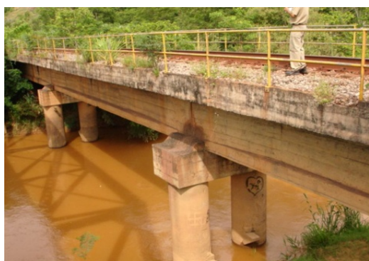
Figure 10 - Oblique view of Suaçui river bridge (2011).
