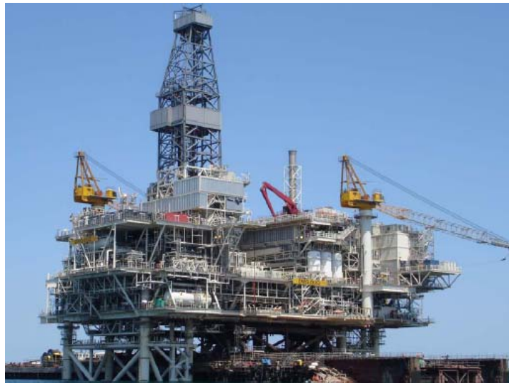
Figura 1. ACG Topsides FloatOver (Topside com 16000t – OTC 19237, 2008)
