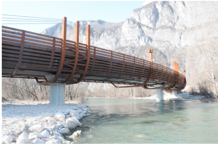
Figure 2. A brand-new COR-TEN bridge structure (Ululone bridge, north of Italy).
