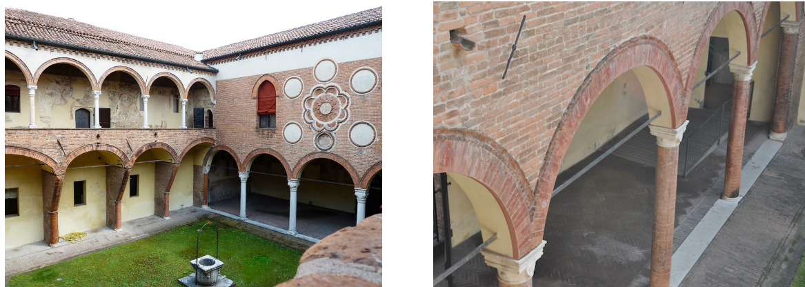
Figure 3. Inner yard of Casa Romei and detail of the ground floor tie-rods.
