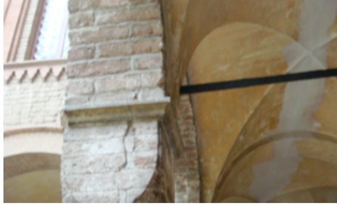
Figure 1. Tie-rod inserting in a masonry column.
