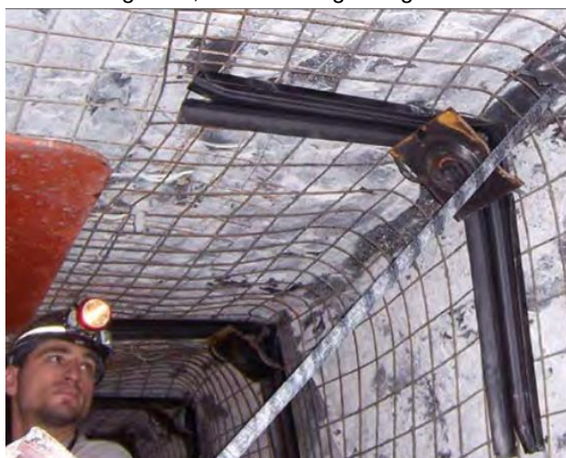
Figure 6 - Recommended support method using bolts, mesh and right-angle-irons.
