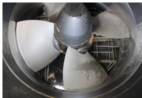
Figure 1: Jirau’s hydropower turbine.
