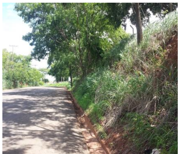
Figura 4. Talude 3 – Campus III da UNESP. Sanches (2015).
