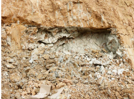
Figure 3. Fissures filling with clay minerals
