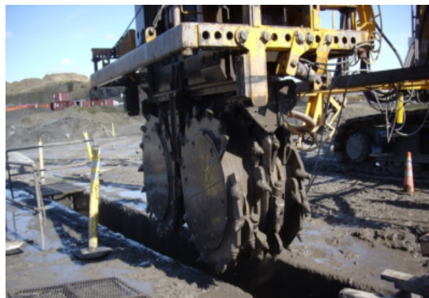
Figure 7. Bauer Cutter Heads Showing RSM Wheel Setup
