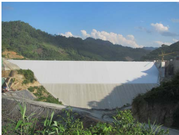
Figure 4. Nam Ou VI GFRD, Stage 2. Waterproofing system completed in 28 days. The geocomposite of Stage 1, covered by dust, looks like concrete.
