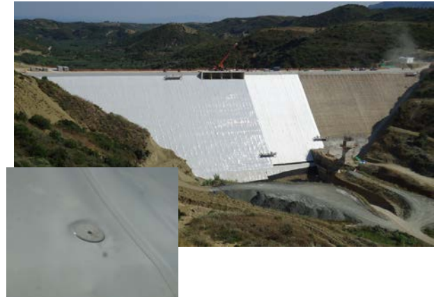
Figure 9. Deep grouted anchors at Filiatrinos hardfill dam. Waterproofing facing completed in one month.
