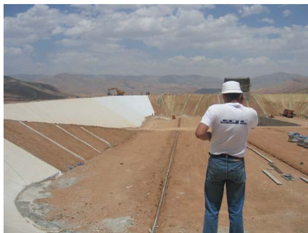
Figure 5. Kohrang dam and headpond, Iran 2004. PVC anchor strips embedded in trenches excavated in compacted soil.
