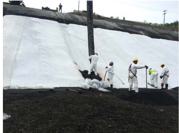
Figure 7. Tensioning anchor trenches at Panama Canal Expansion Water Saving Basins.
