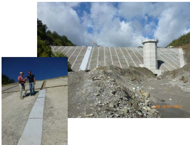
Figure 6. PVC anchor strips embedded in trenches placed between porous concrete slabs at Murdhari GFRD, Albania.
