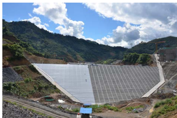
Figure 3. Nam Ou VI GFRD, Stage 1. Dam body and anchor strips completed, PVC geocomposite under installation. Waterproofing system completed in 24 days.
