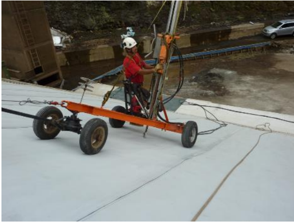
Figure 8. Deep Duckbill anchors at Vaité earthfill dam.
